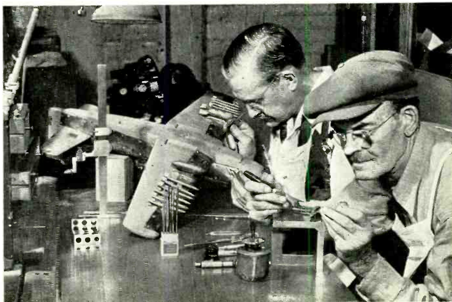
Fig. 7. Scale model aircraft and antenna shown in process of construction. Craftsman in foreground solders a connection in minute cavity type slot antenna. The 1/20th scale aircraft model shown is of wood.
